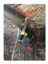
Air Compressor behind the PR3 chamber. · Nomial : on, CARM Lock : off. V Procédure to turn off: Close three values, SW/ off, SW2 to turn on : opposite Way
