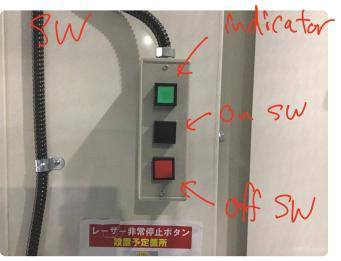
PSL FFU Nominal : On, CARM LOCK : off. . Turn on/off by the circuit breaker on the pillar of the clean booth at the front of PSL room.
