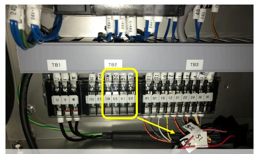
Just in case, we detached the interlock cable of the cooling water circulation system.
